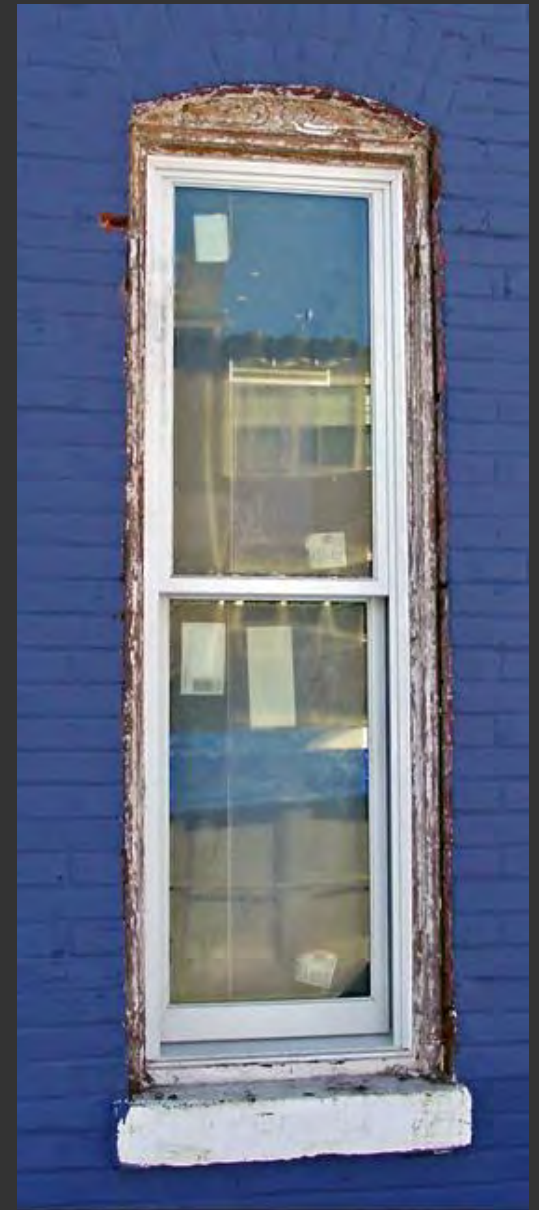
Full RO unit installed within existing jamb
