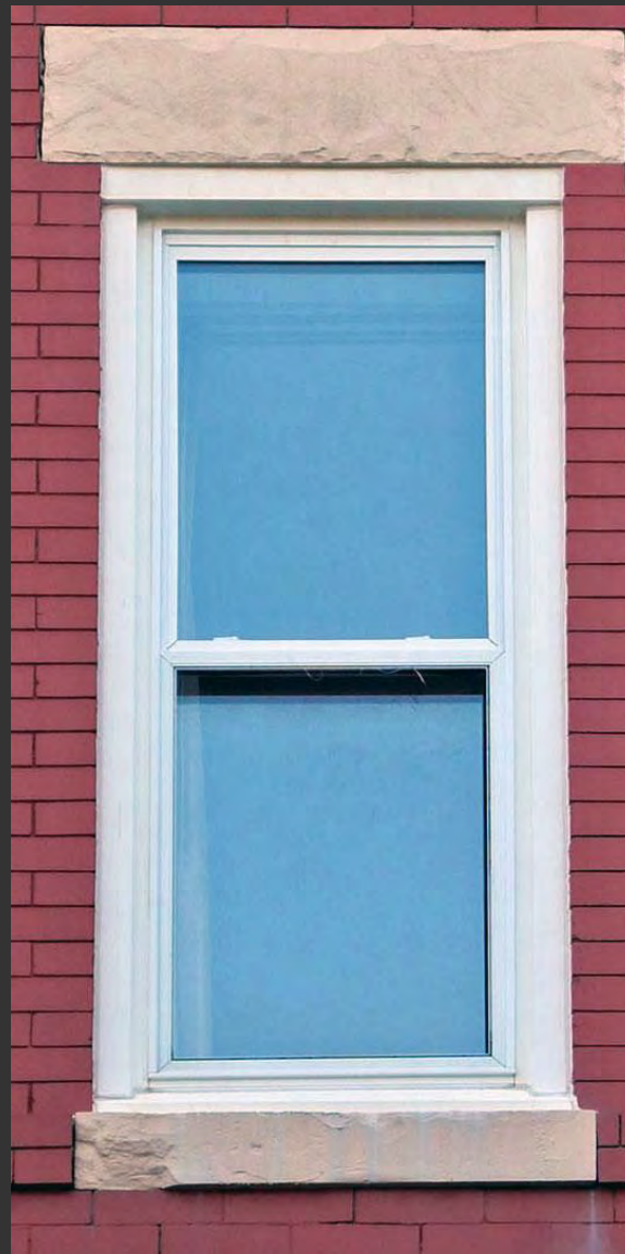
Vinyl windows as typically installed in areas without historic review
