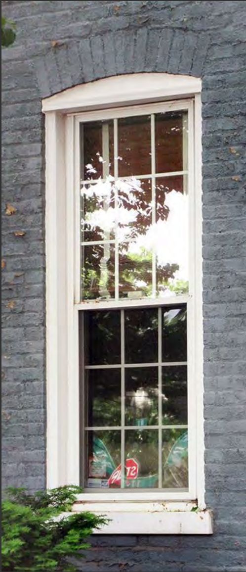
Vinyl windows as typically installed in areas without historic review
