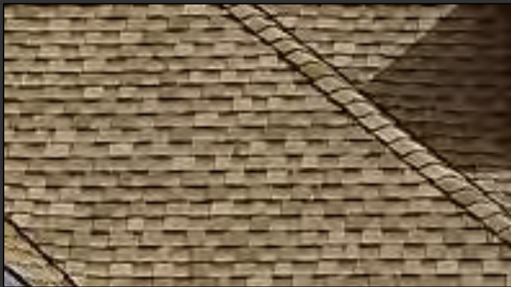
Incompatible architectural fiberglass shingle evoking wood, similar in price to five-tab above
